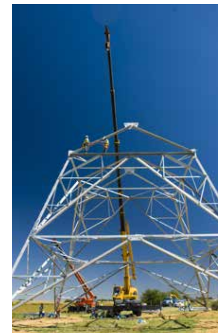
Construction of the Bothaville 765kV line in progress.
