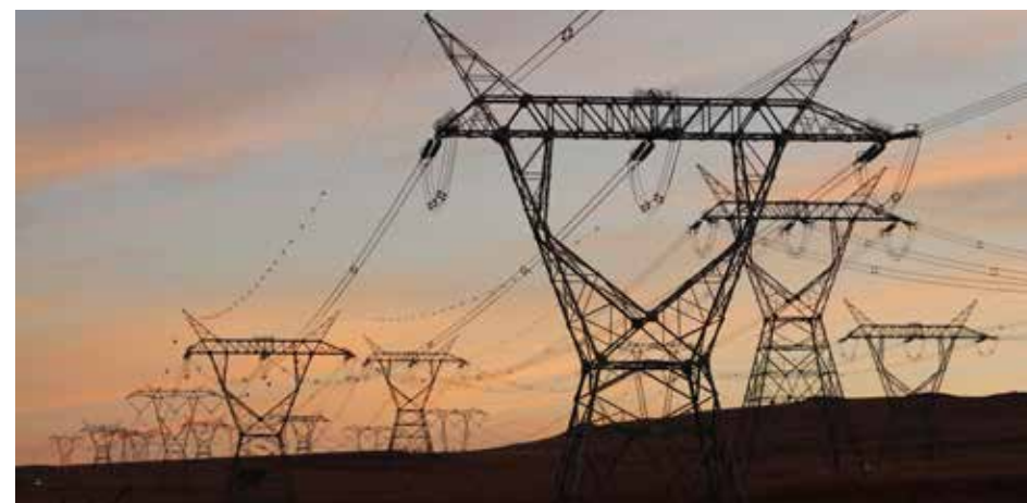
Ingula is connected to the national grid by 400kV Transmission lines. (Photo: Janet du Plooy)
