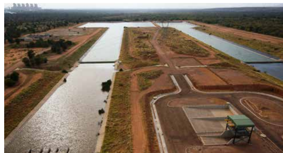
Completion of the Medupi water treatment plant was a key milestone leading up to synchronisation and commissioning of Unit 6. Matimba Power Station is visible in the background.
