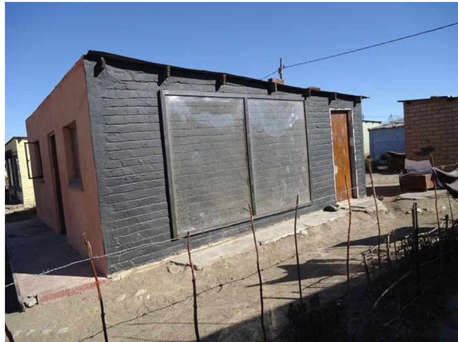
Full thermal insulation: ceilings + three insulated walls + Trombe wall
