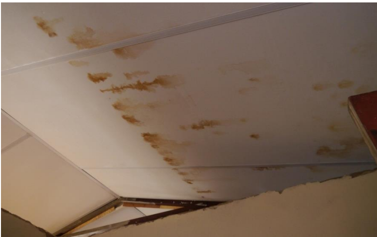
Figure 6: Brown marks on the ceiling as a result of roof leaks.
