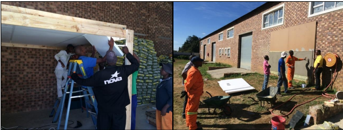
Figure 5: Member of the newly appointed team being trained on the installation of insulation at the storage facility near KwaZamokuhle.
