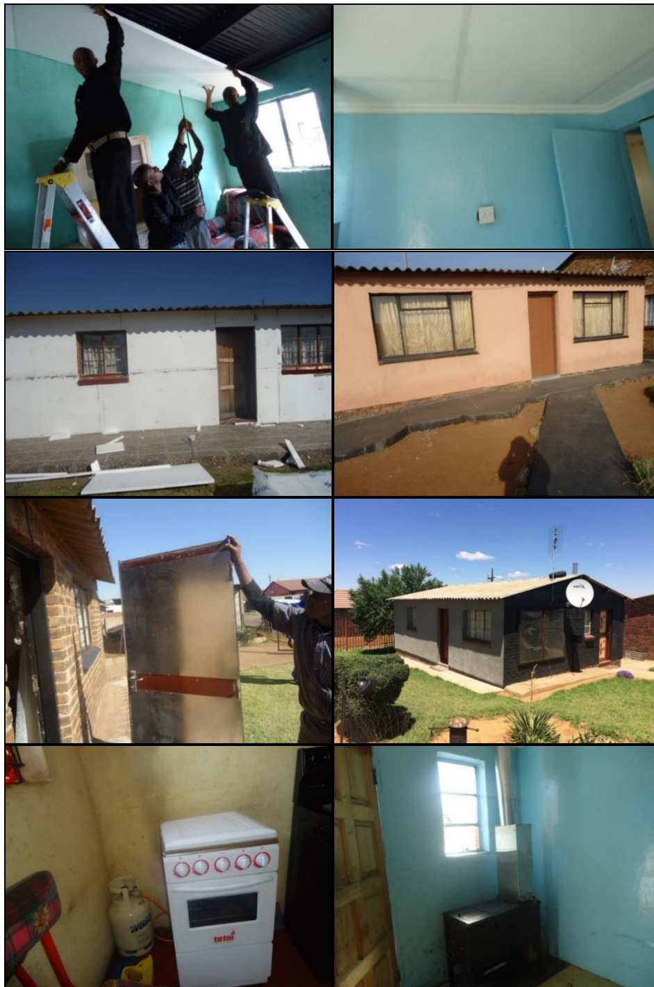
Figure 9: Images of the installation process, completed thermal installations and stove replacements
