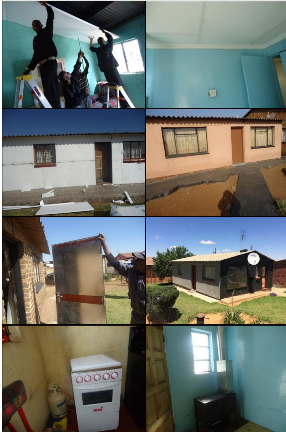
Figure A8: Images of the installation process, completed thermal installations and stove replacements
