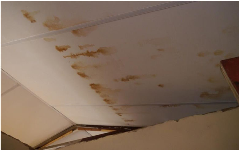
Figure A6: Brown marks on the ceiling as a result of roof leaks.
