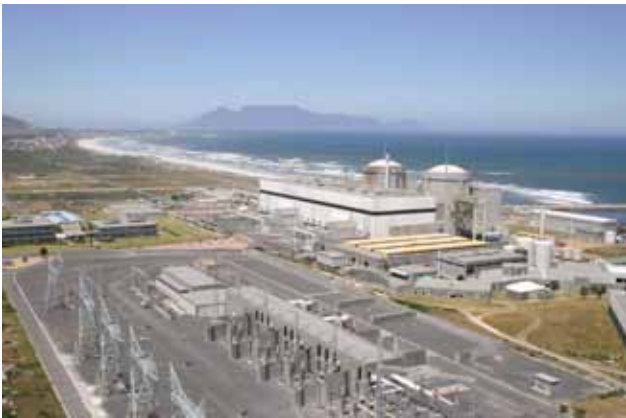
Koeberg power station near Cape Town
