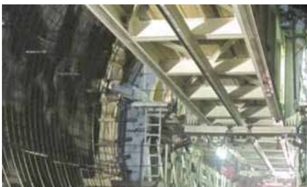
Ingula: Low pressure headrace tunnel 3 and 4 full round shutter
