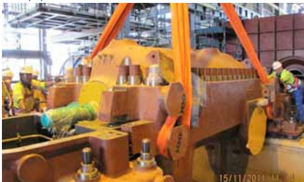
HP (high pressure) turbine installation at Medupi power station, November 2011
