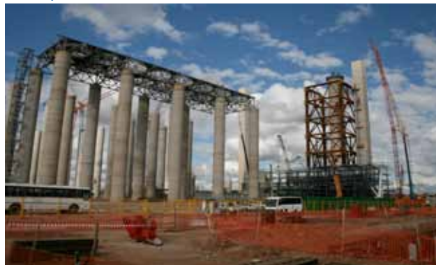
Kusile boiler erection, November 2011
