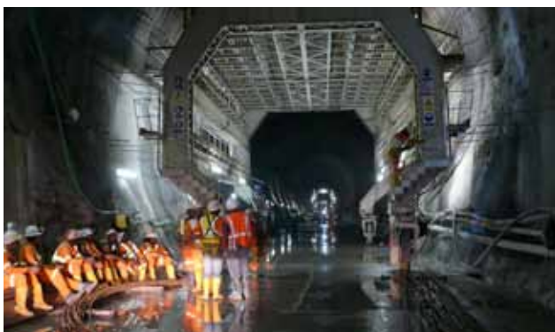
All tunnels for the Ingula pumped storage scheme have been completed
