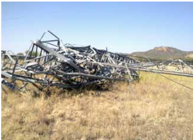
Pylon theft is becoming a major problem for Eskom
