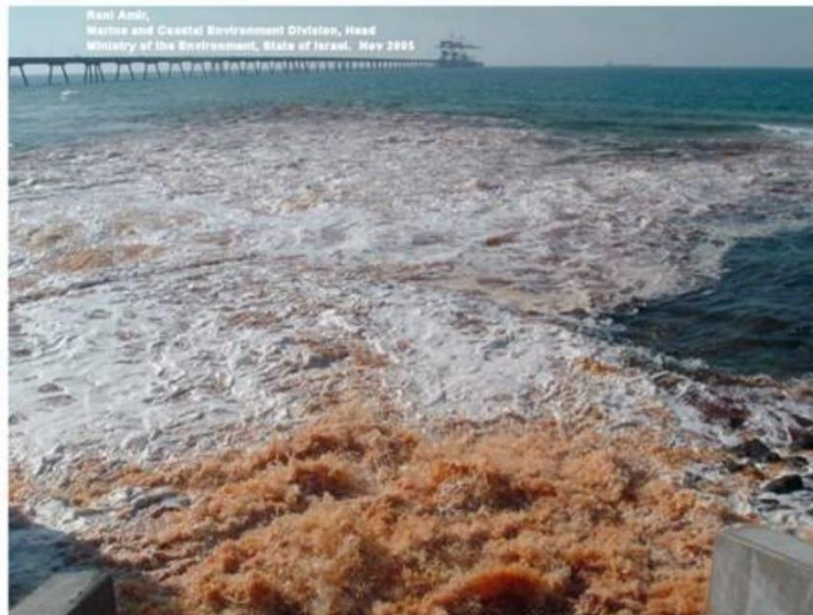
Figure 4.23: Brine discharge from a reverse osmosis desalination plant employing ferrous sulphate as a coagulant in intake water pre-treatment. The red colour is due to particulate ferric hydroxide discharged in the brine effluent (from UNEP 2008).
