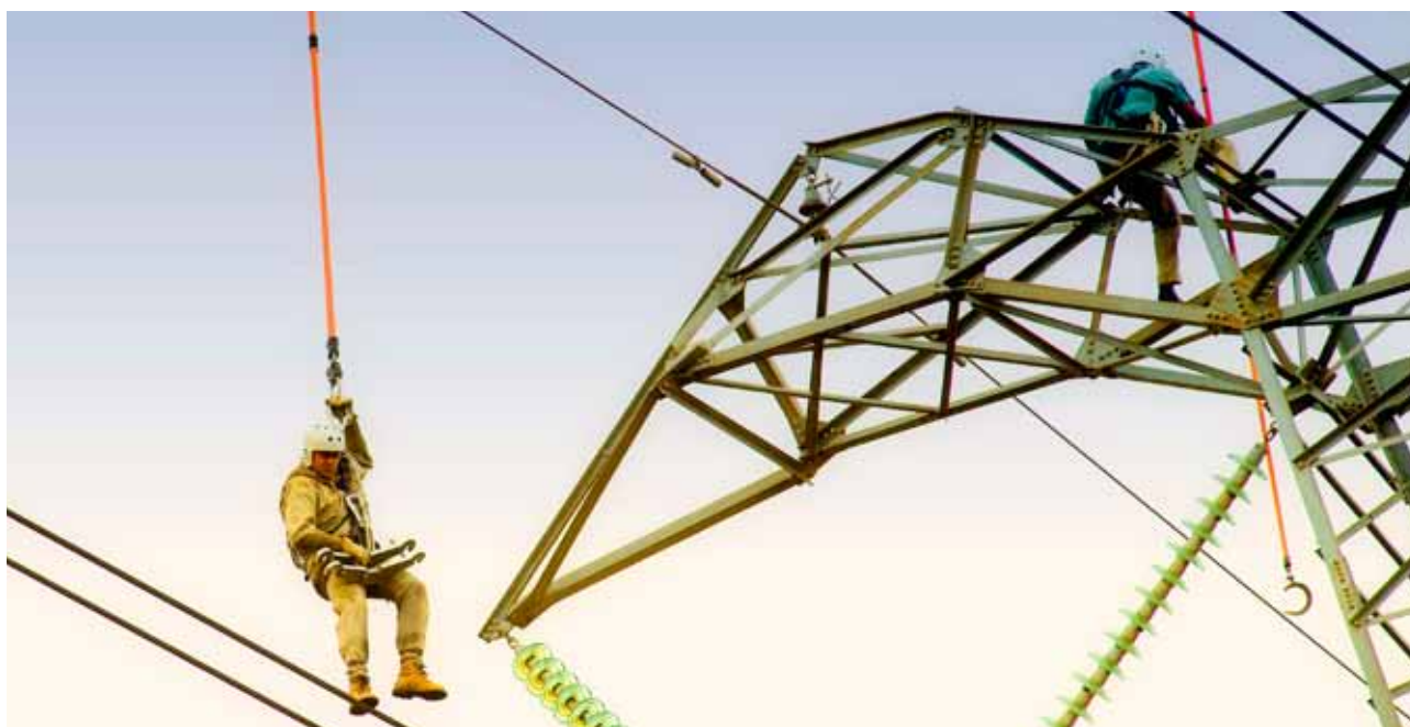
Liveline maintenance work reduces downtime on networks.
