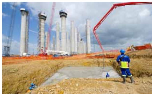
Kusile power station.
