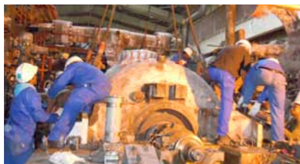
The damage to the 600MW unit 4 at Duvha power station is being assessed and the clear-up operation is in progress.
