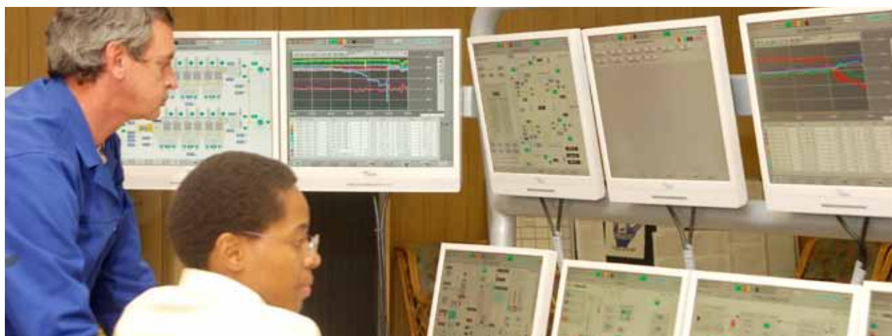
Unit operators run power station control rooms 24 hours a day.
