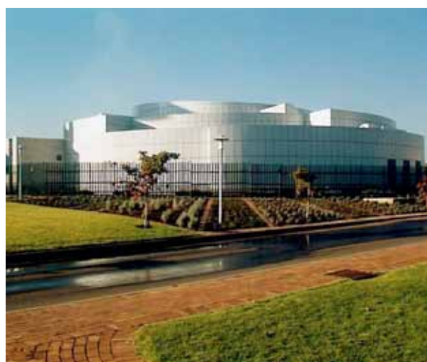
National control centre in Simmerpan, Johannesburg.
