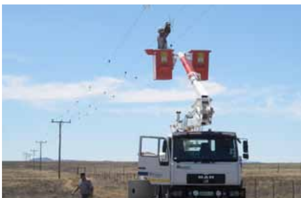
Bird diverters were strung on a high-voltage line in the Karoo to prevent bird fatalities.
