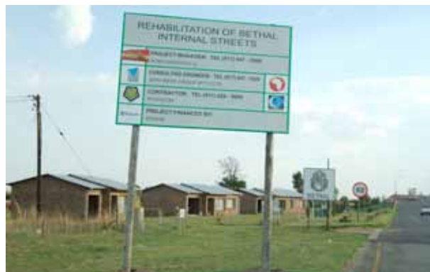
Road repair project in Bethal.
