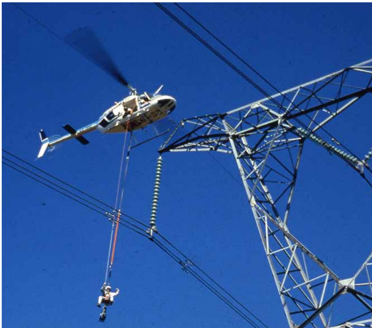
Liveline teams maintain high-voltage lines under live conditions to reduce inconvenience to customers.
