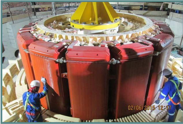
Rotor being lowered into stator
