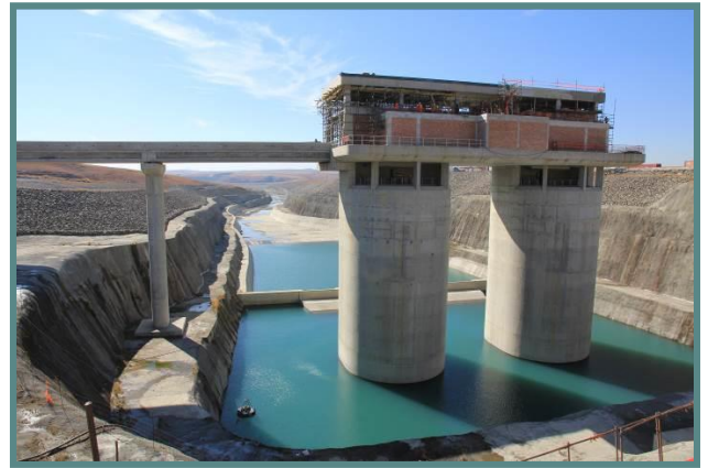
Intake canal and headrace
