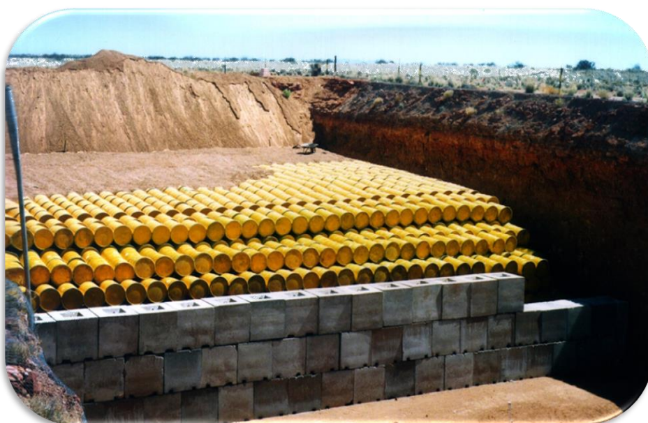
Drums containing low-level waste are covered with a layer of clay and then top soil.
