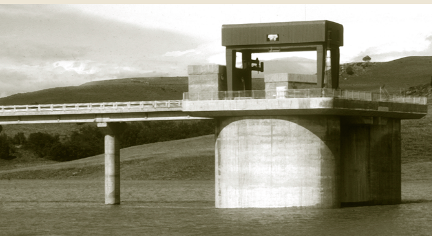
THE 6 m HEADRACE INLETS, SITUATED IN THE DRIEKLOOF DAM, HOUSE THE EMERGENCY / MAINTENANCE GATES
