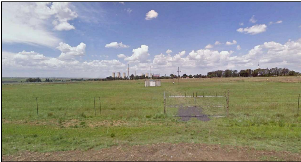
Figure 8-47: View of the PV Site B from the west
