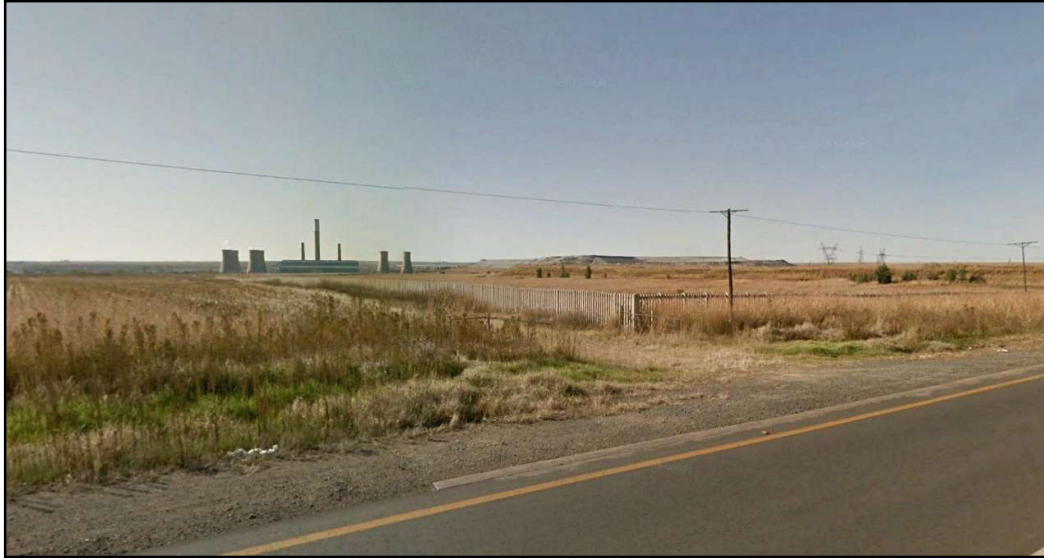
Figure 8-46: View of the PV Site A from the R542 arterial road (LOGIS, 2022)
