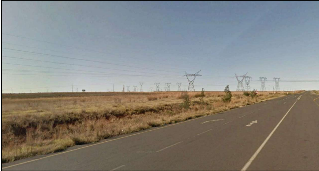
Figure 8-50: Power lines near the R542 arterial road
