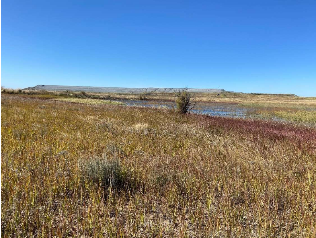
Figure 8-38: Ash dam facility and pooling of water at dam
