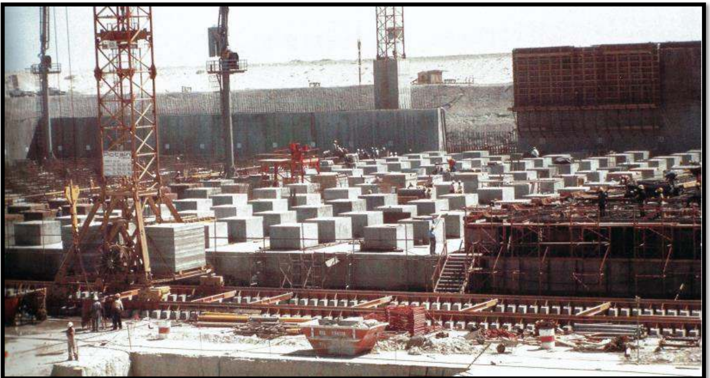
Above: 676 reinforced concrete pedestals for 1 829 seismic bearings under construction in 1978
