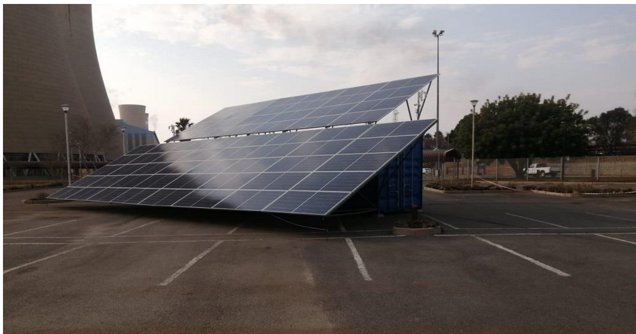
Picture 8.1: A containerised microgrid at KPS
