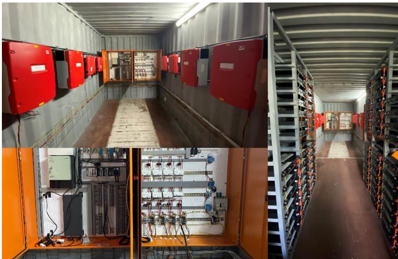
Picture 8.2: Control and communication systems and lithium-ion battery banks inside the container
