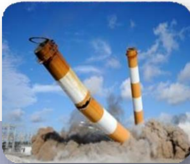
Component A: Decommissioning
