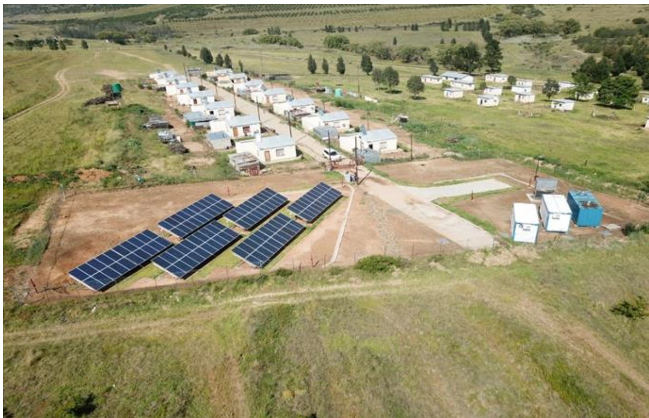
Picture 8.3: Ficksburg microgrid
