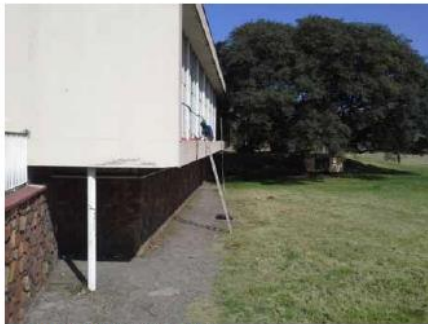
REAR AREA OF BUILDING
