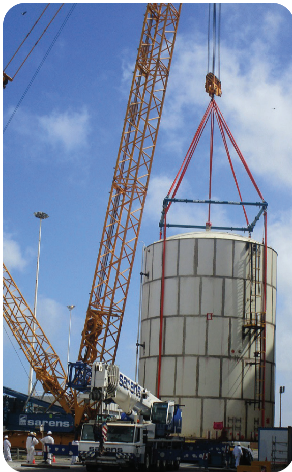
I-Reactor Cavity kunye neTanki yeNkqubo yokuPholisa i-Fuel Pool.
