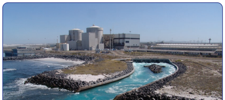
The Koeberg Nuclear Power Station intake basin and outflow of cooling water from the Atlantic Ocean. This type of cooling saves South Africa more than 2 billion litres of water per year.
