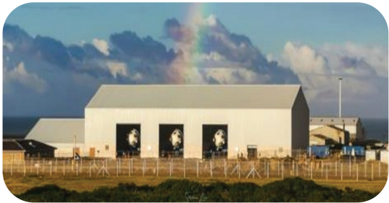
The storage facility housing the replacement steam generators.
