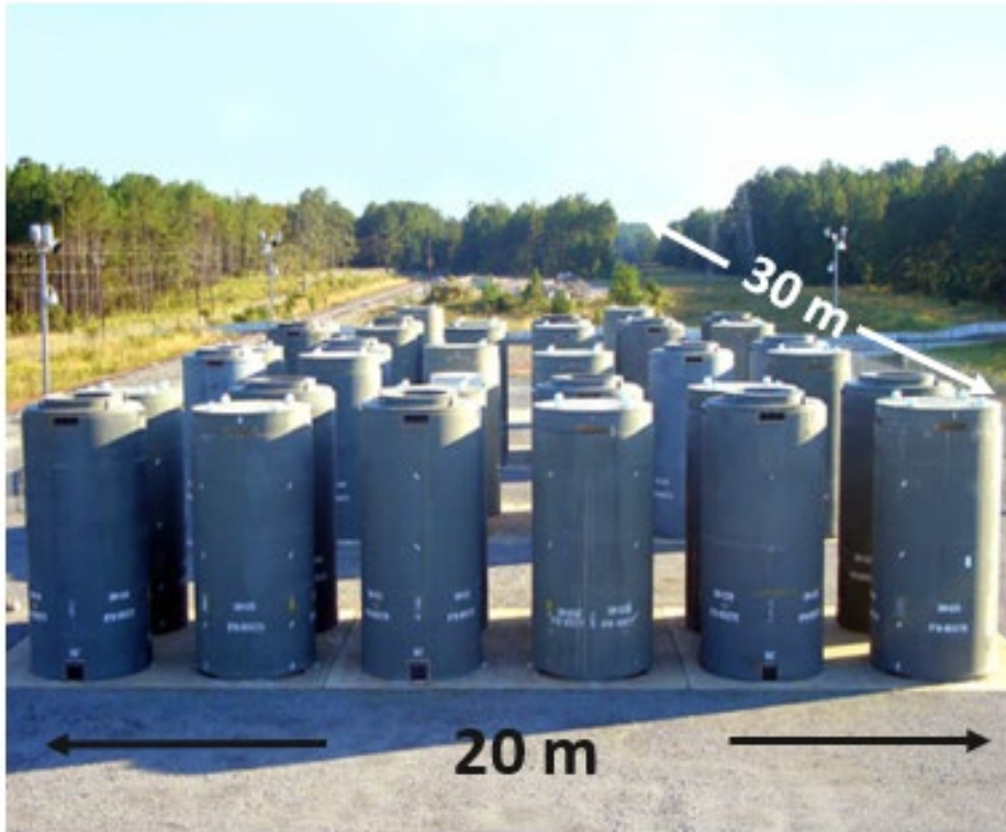
Figure 17: An example of a dry cask storage area for spent nuclear fuel
