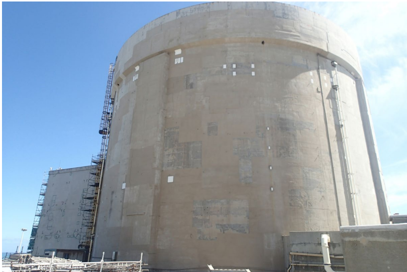
Figure 5: The Koeberg containment building
