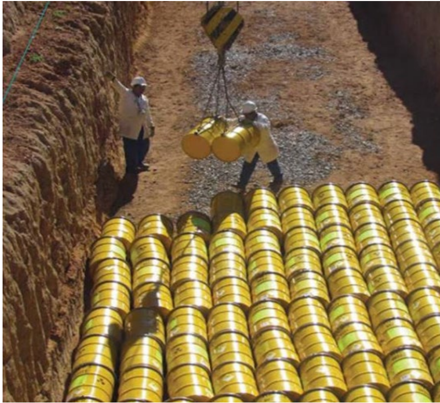
Figure 11: Radioactive waste in steel drums stored at Vaalputs National Waste Disposal Facility
