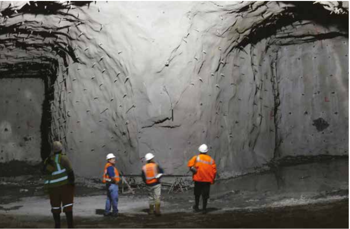
LEFT: Reinforcing the bifurcation (splitting into two) of the tailrace tunnel PHOTO BY DU FILMS
