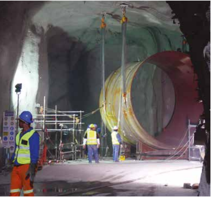
BOTTOM RIGHT: Steel linings being installed PHOTO BY FIFI MEYER
