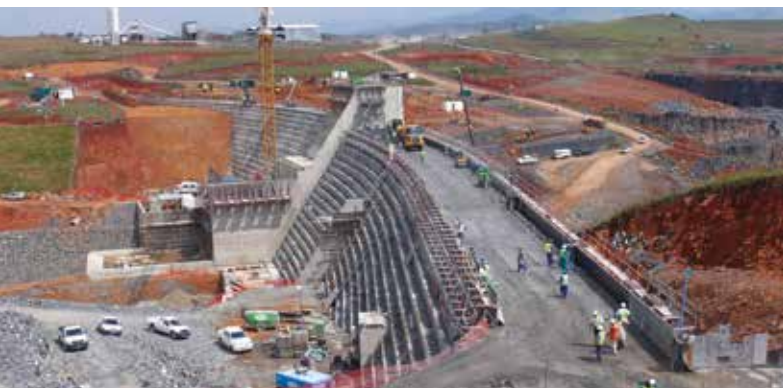
TOP LEFT: Layers of roller-compacted concrete being placed on Bramhoek Dam's wall
