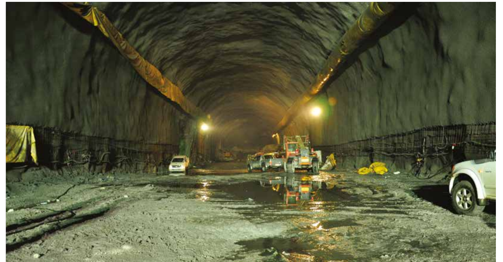
BELOW: Progressive downward excavation of the machine hall
