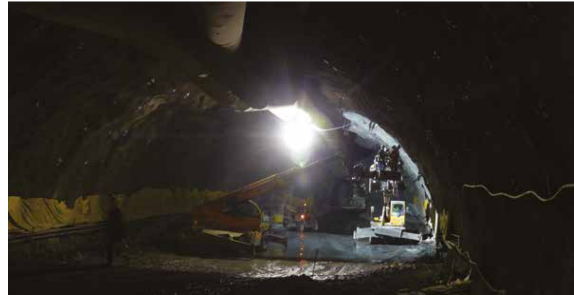
TOP: Initial excavations of the transformer hall ceiling
