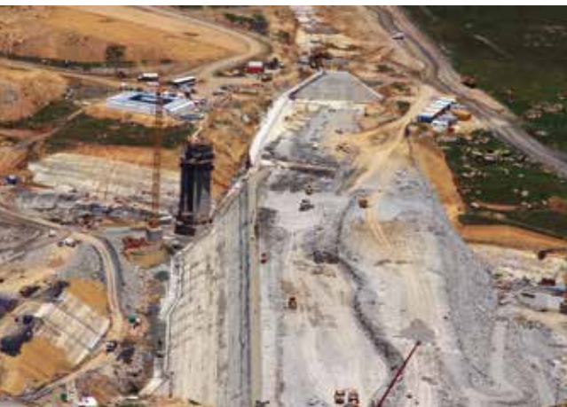
FROM LEFT: Progress on the Bedford sandstone rock-fill dam, with only an up-stream concrete lining
