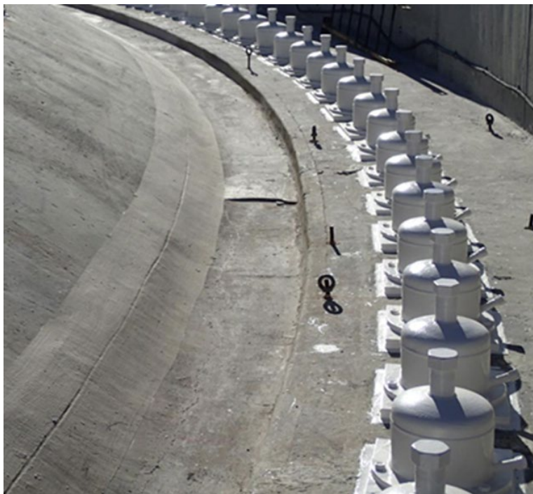
Figure 8: Containment dome crack sealed and coated
