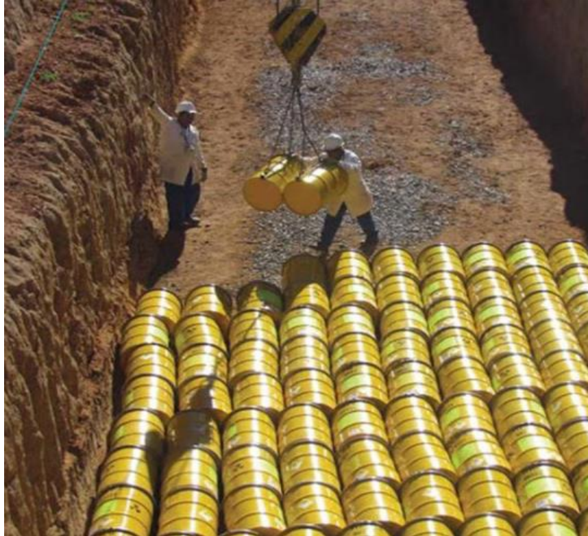
Umfanekiso 11: Inkunkuma yerhasi esebenzayo kwimigqomo yentsimbi egcinwe Kwiziko Likazwelonke Lokulahla Inkunkuma (National Waste Disposal Facility) Vaalputs
