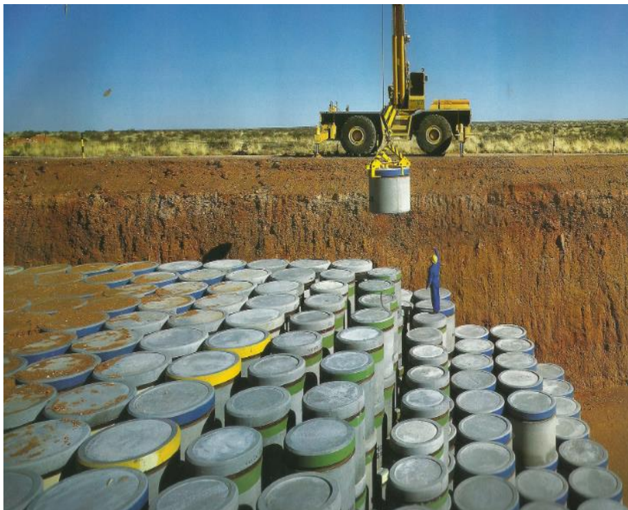
Umfanekiso 12: Inkunkuma yerhasi esebenzayo igcinwe kwimigqomo yekhonk'rithi Kwiziko Likazwelonke Lokulahla Inkunkuma (National Waste Disposal Facility) Vaalputs
