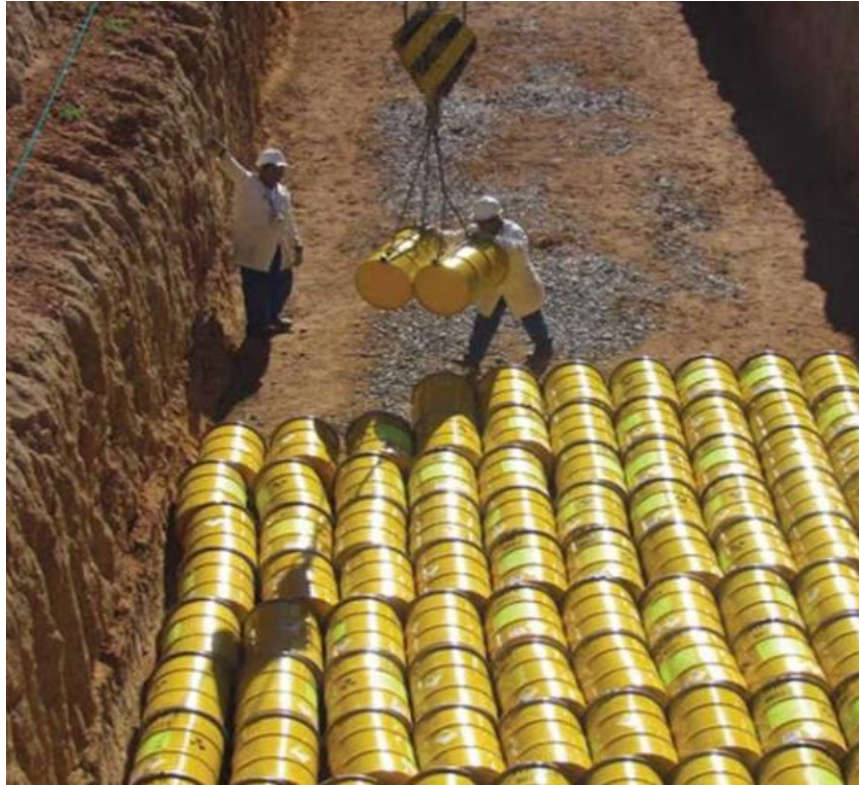
Setshwantsho 11: Matlakala a a nang le marang a a kotsi a a mo teng ga dikgamelo tsa tshipi a a bolokilweng kwa Lefelong la Bosetšhaba la go Latlha Matlakala Kwa Vaalputs
