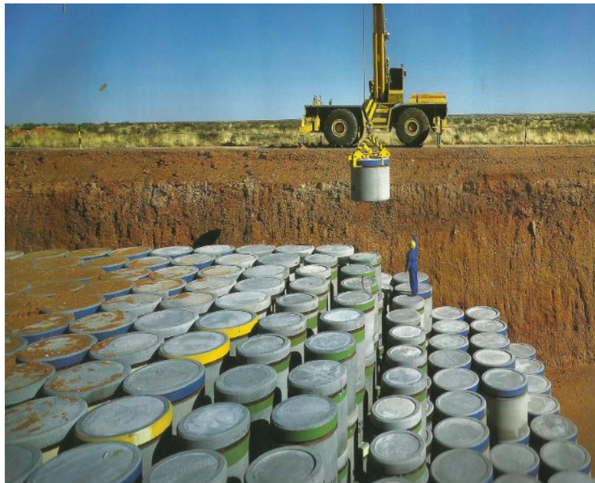
Setshwantsho 12: Matlakala a a nang le marang a a kotsi a a mo teng ga kgamele ya konkoreite e e bolokilweng kwa Lefelong la Bosetšhaba la go Latlha Matlakala la Vaalputs
