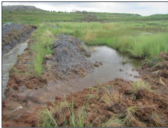
Figure 8-40 - Drainage channels that have been excavated by power station management to prevent the flooding of access roads
