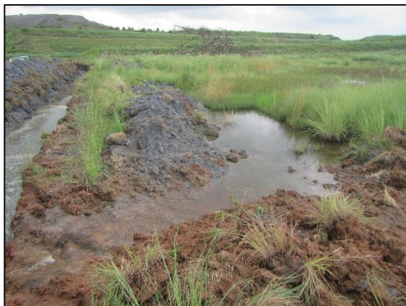
Figure 18: Drainage channels that have been excavated by power station management to prevent the flooding of access roads.
