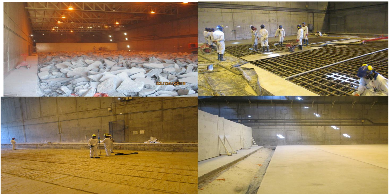
Figure 6: Reinforcement of the CSB Storage Pad
