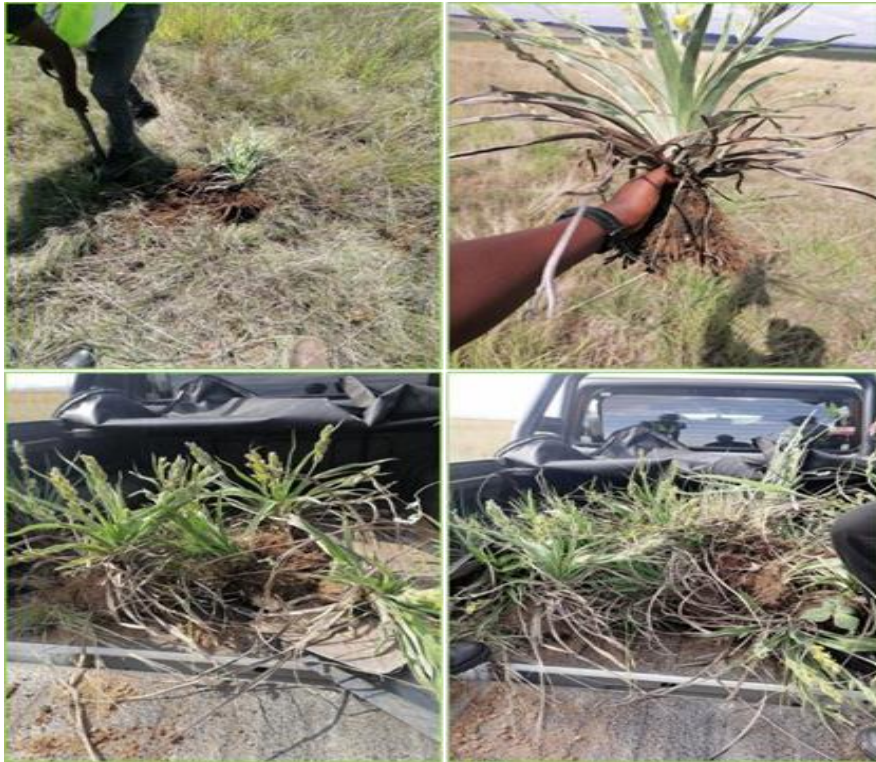
Figure 3-4: Removal and transportation of plant species into the relocation area.
