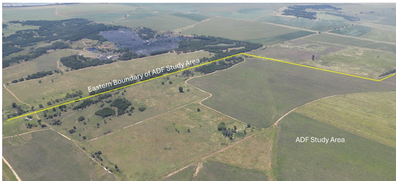
Figure 9: Aerial photograph of the ADF study area viewing the eastern boundary, taken by drone in May 2024.
