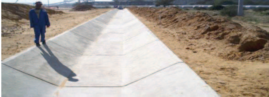
Figure 22: Finished Trapezoidal Drainage Channel
