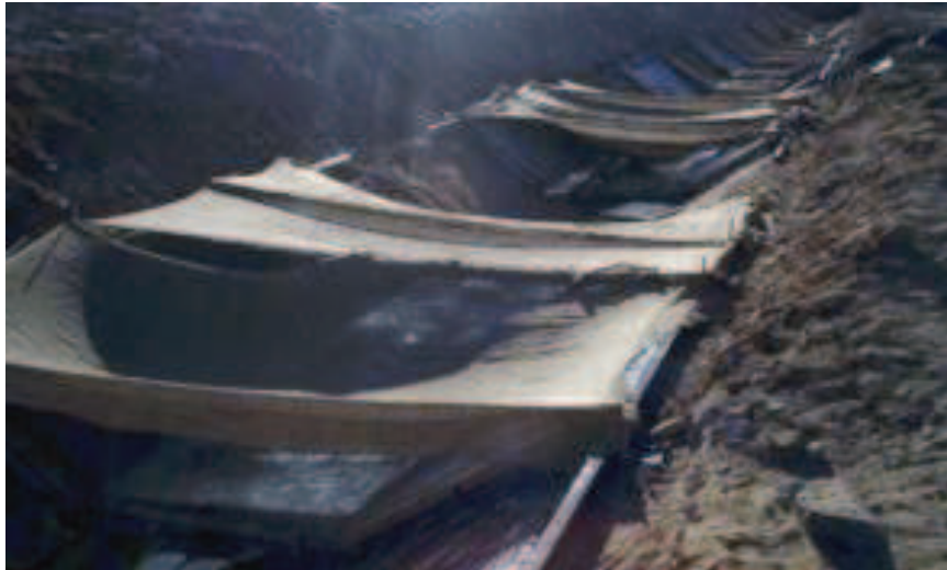
Figure 21: Trapezoidal Drainage Channel Curing
