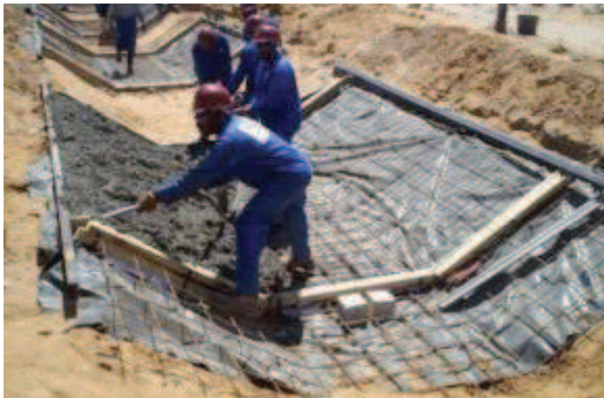
Figure 20: Trapezoidal Drainage Channel Concrete Pouring in Alternating Panels
