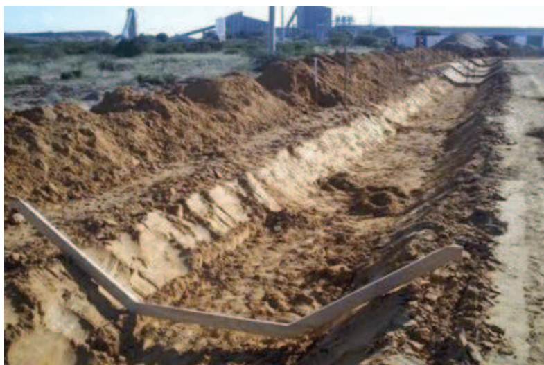
Figure 17: Bulk Excavation of Trapezoidal Drainage Channel
