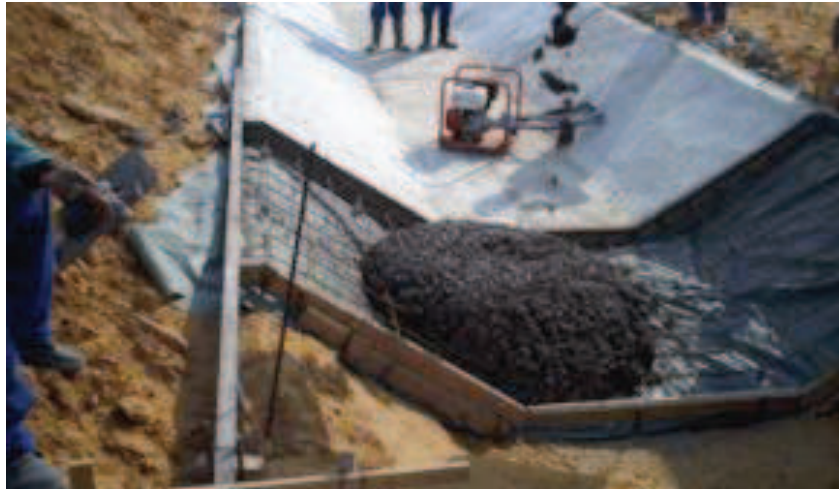
Figure 19: Trapezoidal Channel Concrete Pouring
