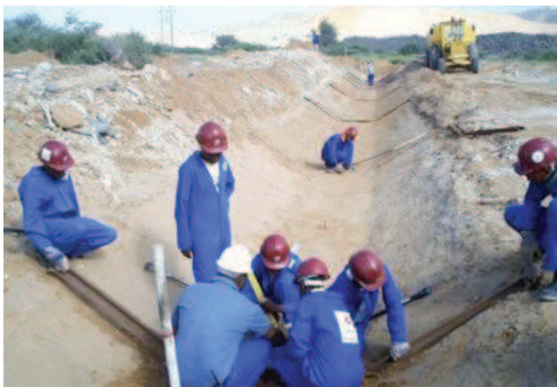
Figure 18: Excavation to the Correct Profile
