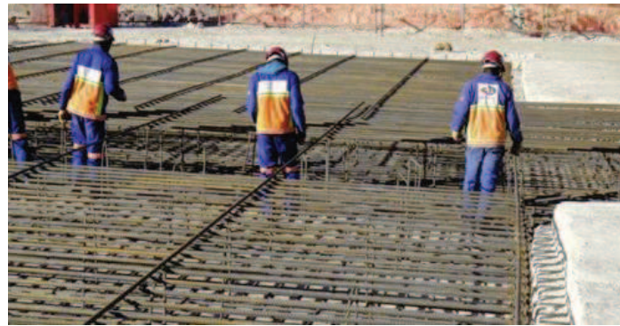
Figure 14: Rebar Fixing
