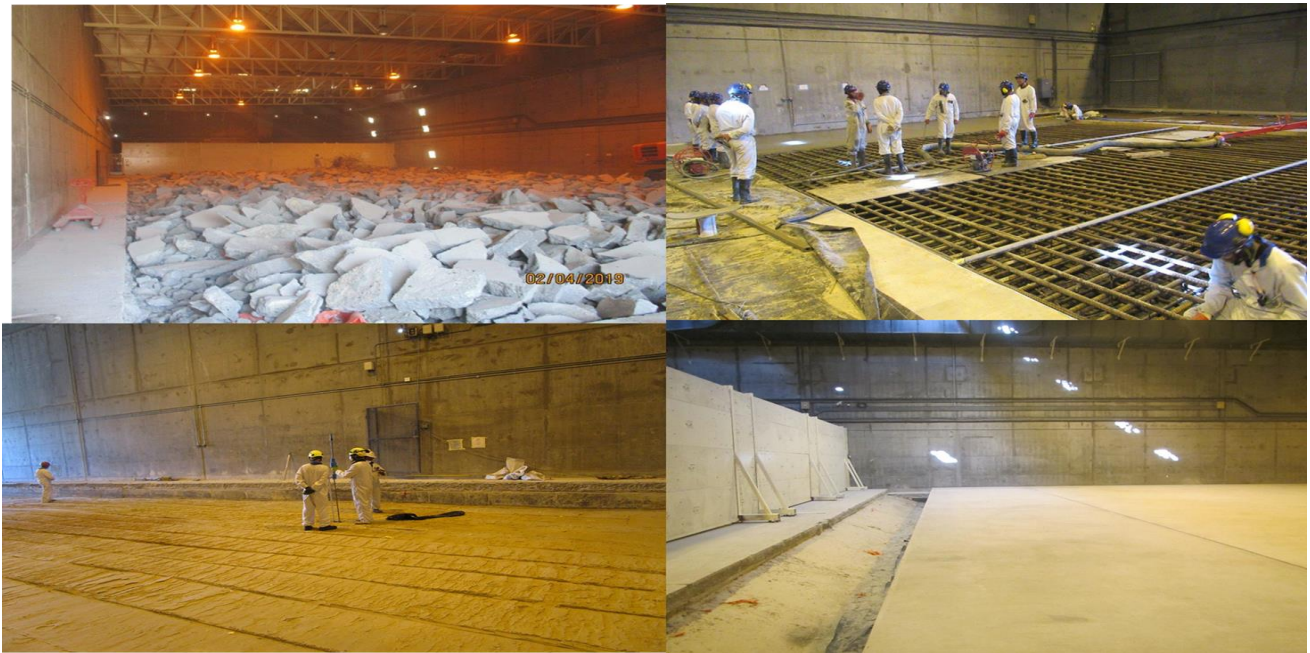
Figure 6: Reinforcement of the CSB Storage Pad
