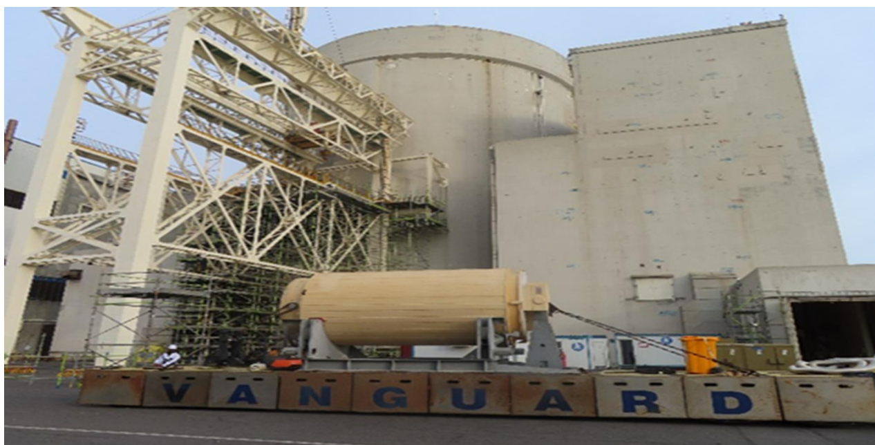
Figure 4: Transfer of a Loaded HI-STAR 100 Cask from the Fuel Building to the CSB
