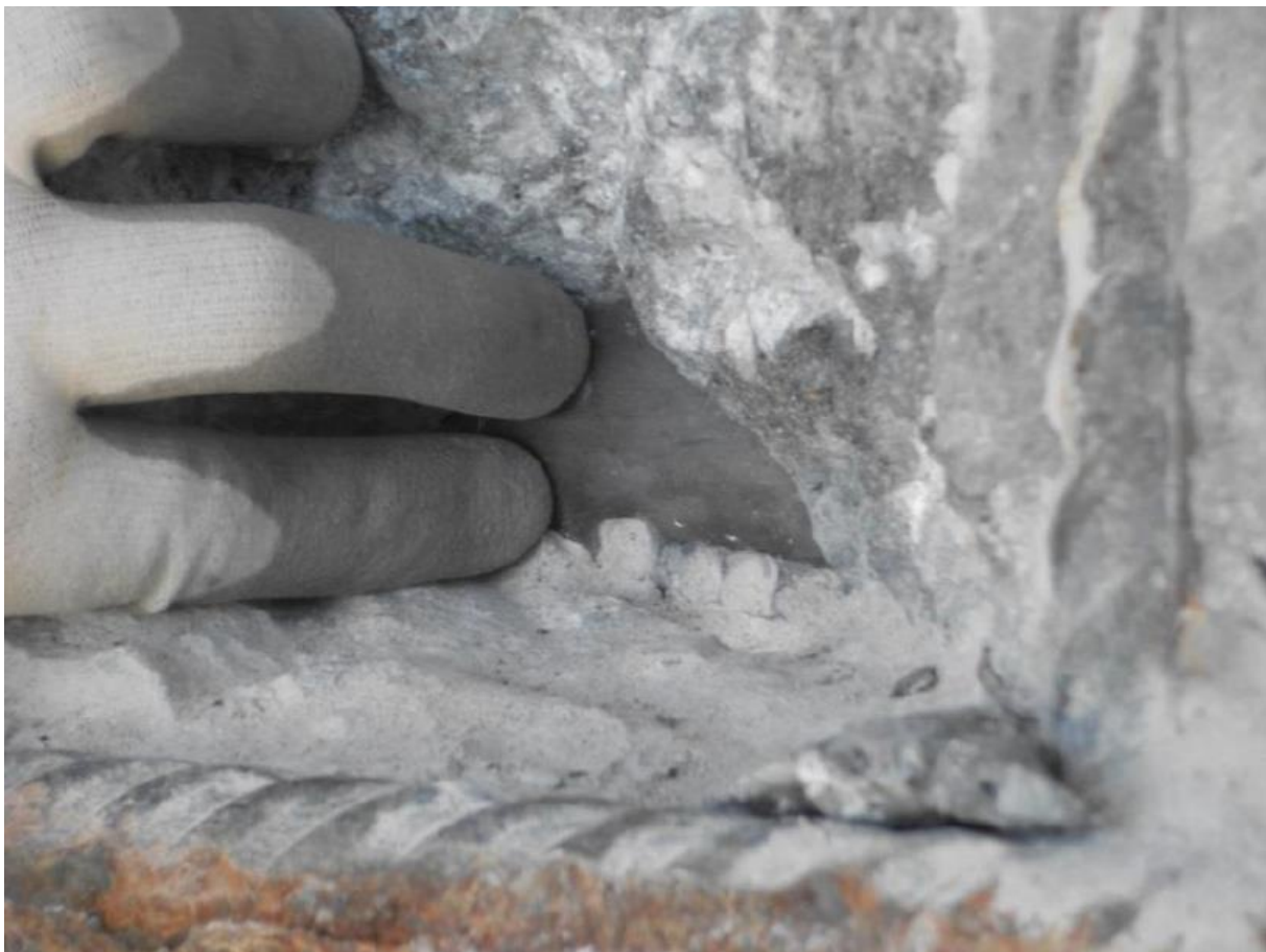
Figure 68: Exposed Tendon Duct
