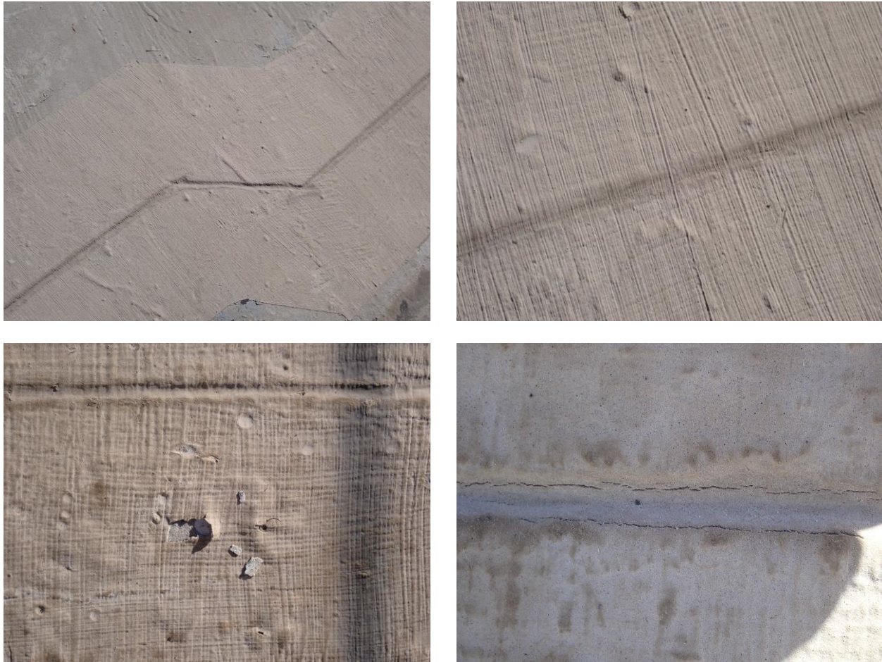
Figure 75: Condition Assessment of Repaired 1 HRX Dome Crack
