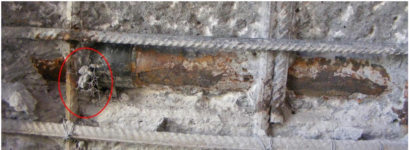
Figure 69: Corroded Duct (Cold Joint)
