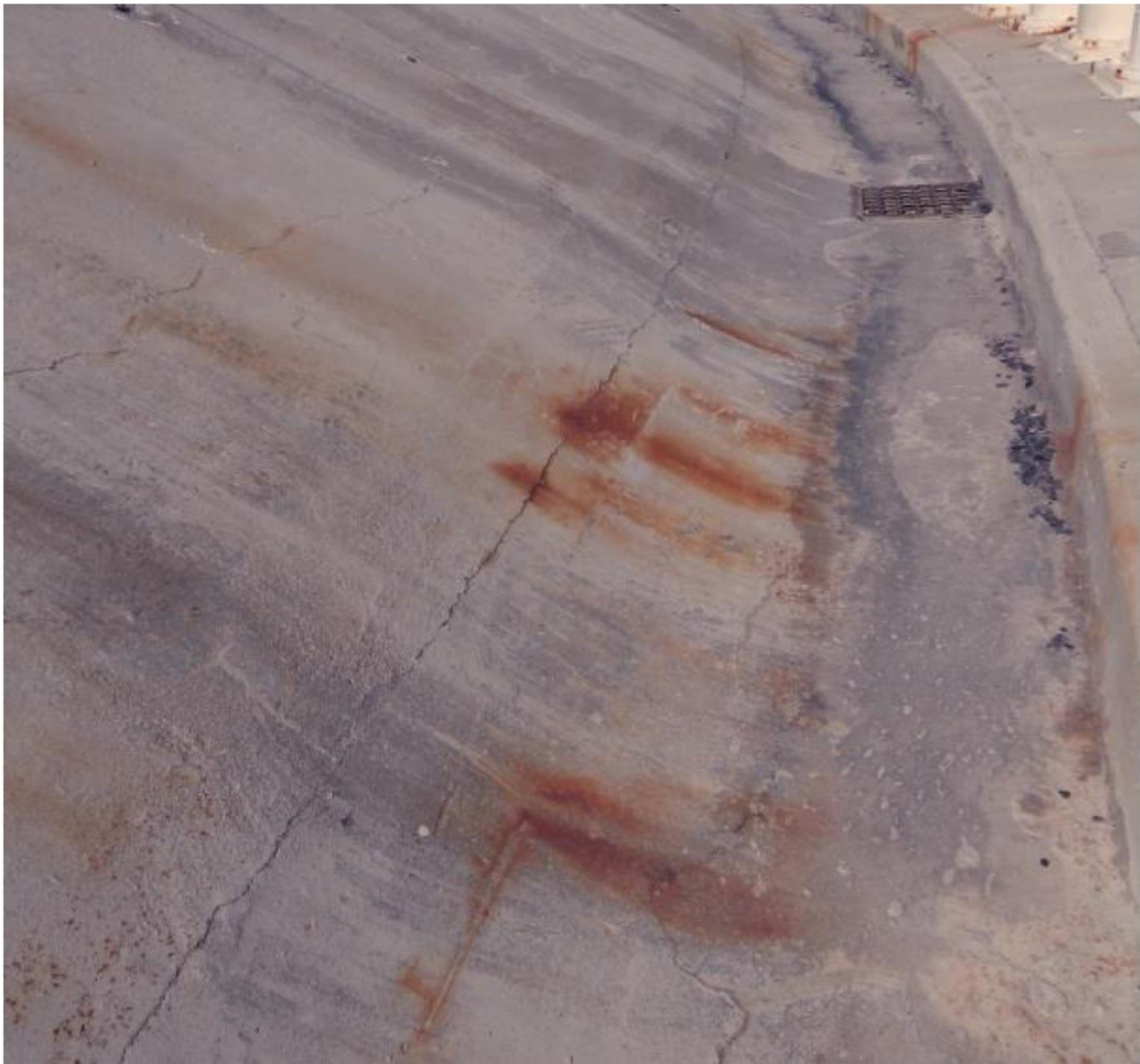
Figure 72: Crack on Domes
