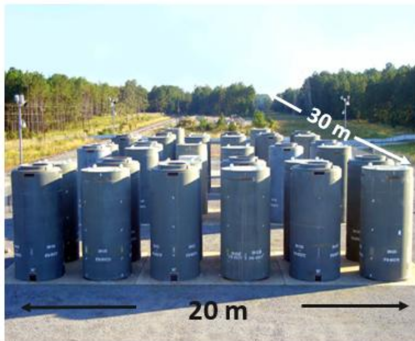
Figure 16: An example of a dry cask storage area for spent nuclear fuel
