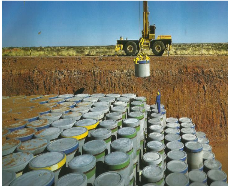
Figure 11: Radioactive waste in concrete waste drums stored at Vaalputs National Waste Disposal Facility
