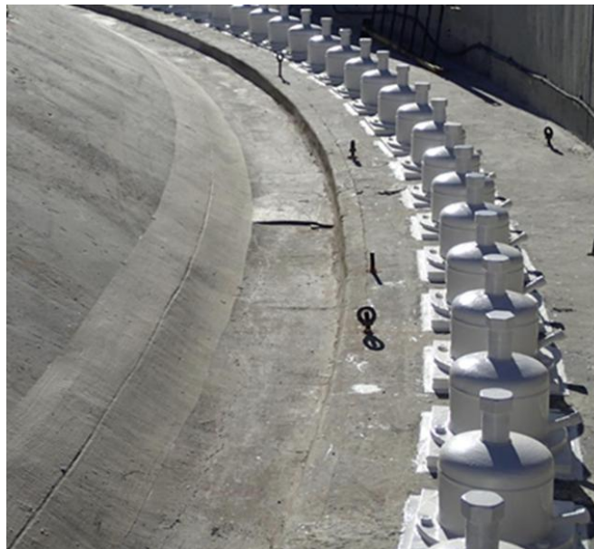
Figure 8: Containment dome crack sealed and coated
