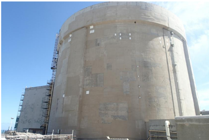
Figure 5: The Koeberg containment building
