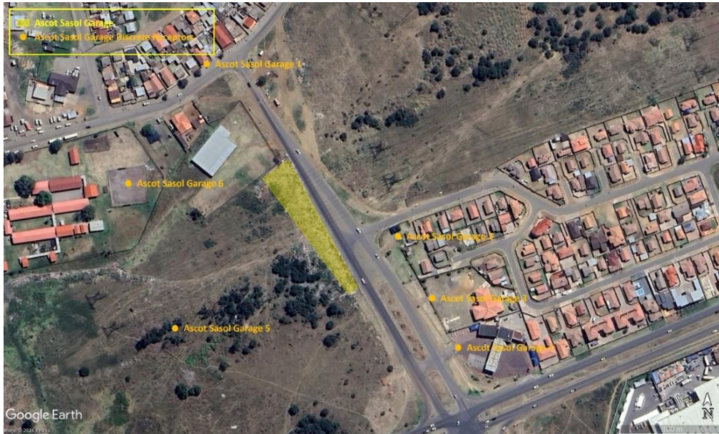
Figure 4-139: Ascot Sasol Garage waste burning site and sensitive receptors near the site.
