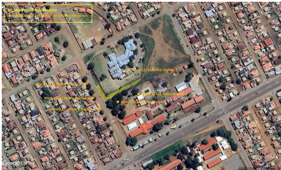
Figure 3-32: Ward 12/13 Police Station waste burning site and sensitive receptors near the site.
