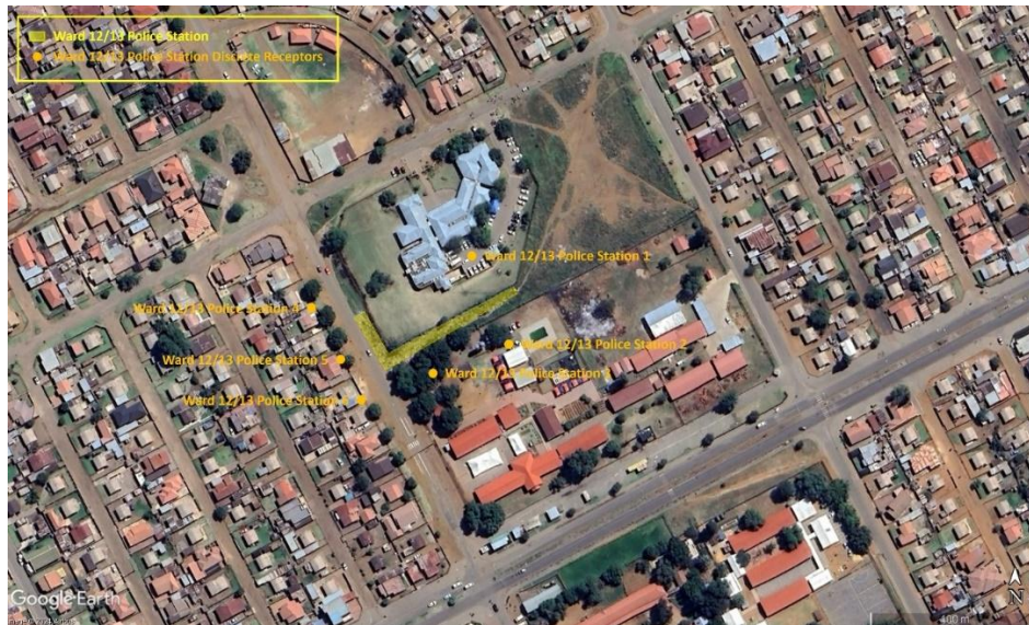
Figure 4-58: Ward 12/13 Police Station waste burning site and sensitive receptors near the site.
