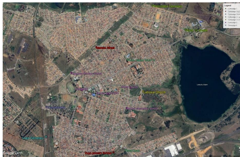
Figure 7: Location of the illegal waste sites that Eskom has cleaned up to date
