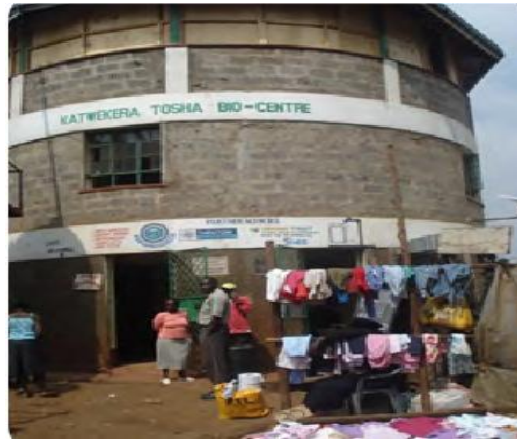
Figure 11 A Bio-sanitation facility at Katwekera village, Kibera
