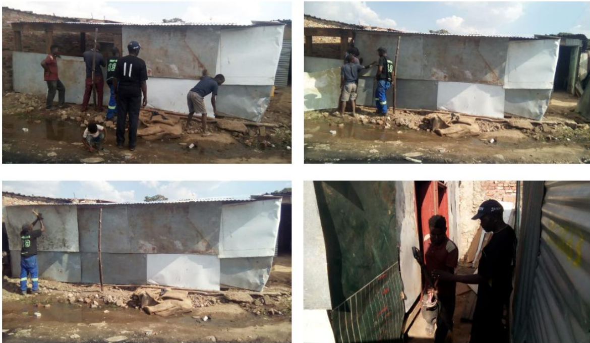
Figure 6: Construction of an Informal House in Zandspruit (Stevens D 2019)
