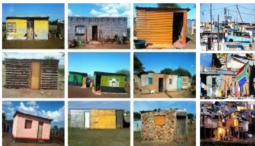
Figure 4 Structure of Informal Houses
