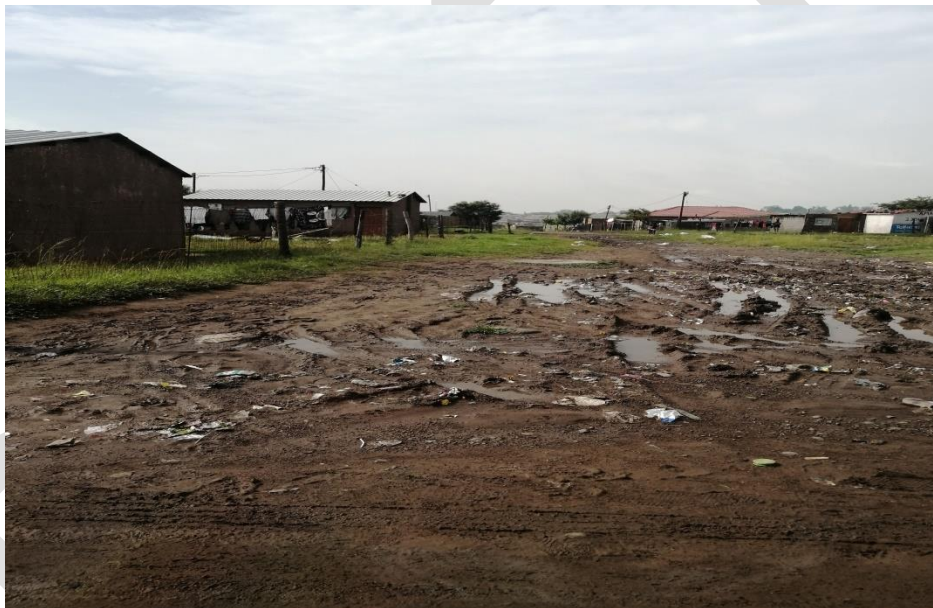
Figure 11: Road conditions in Ezamokuhle
