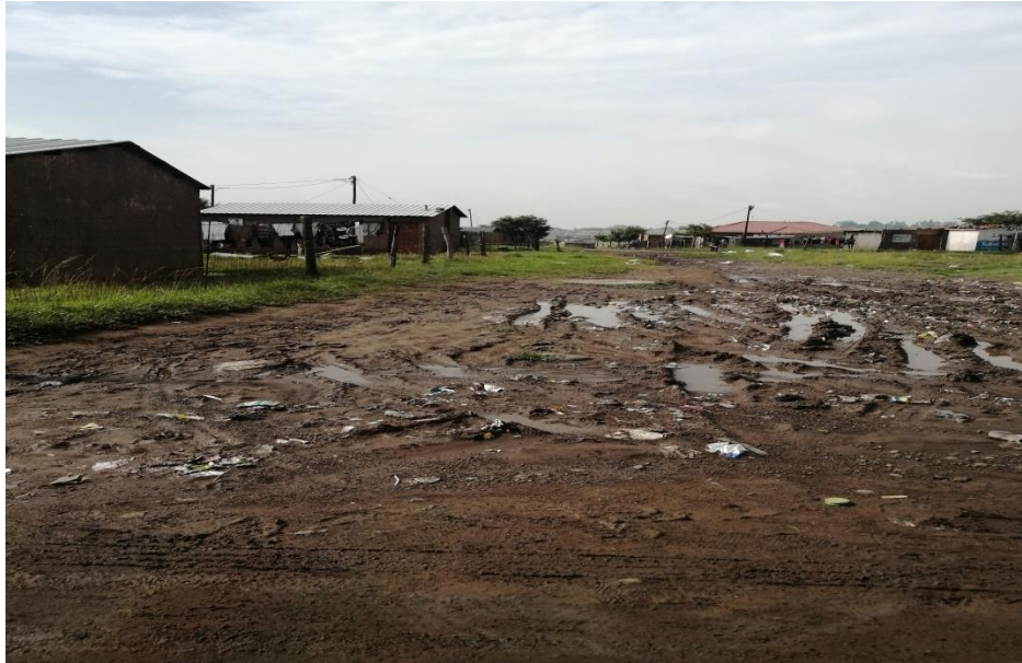
Figure 12: Road conditions in Ezamokuhle
