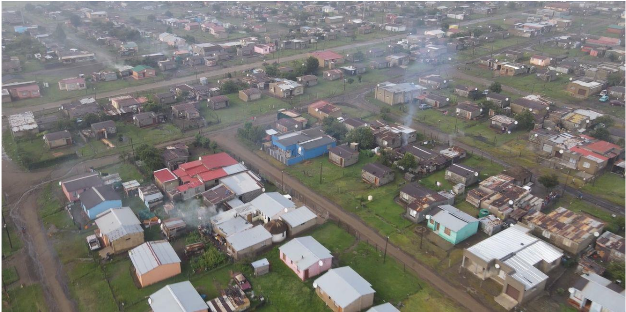
Figure 28: Satellite dish connections to households
