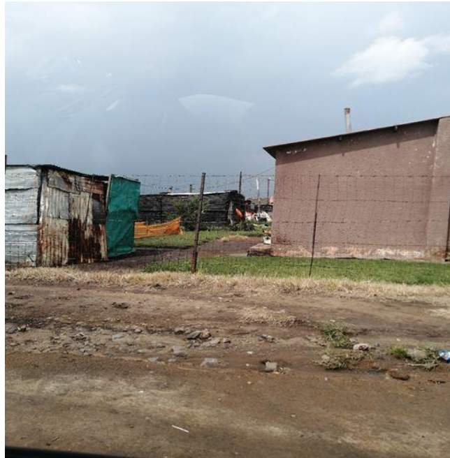
Figure 30: Electricity connection between RDP housing and informal household
