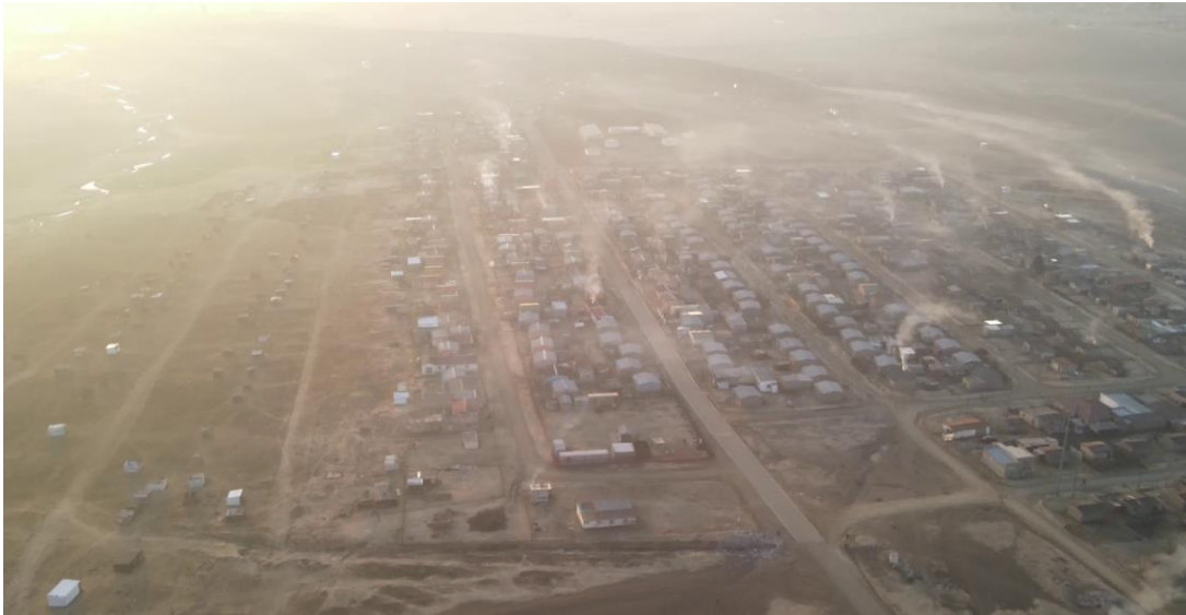
Figure 46: Ezamokuhle unpaved inner roads from aerial survey
