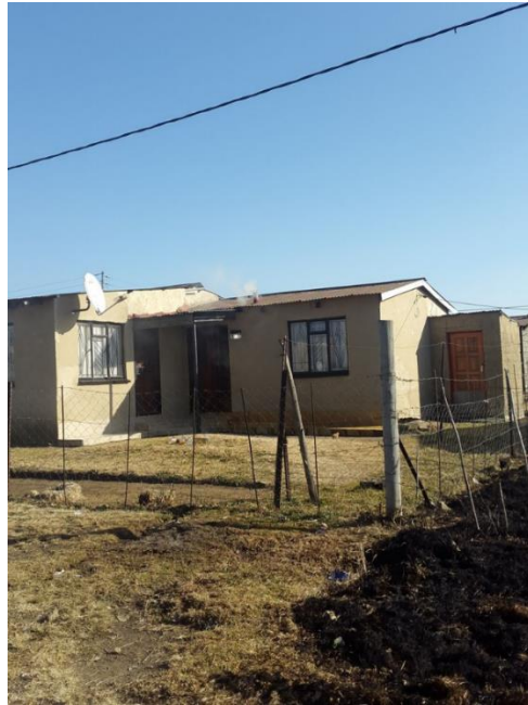
Figure 34: Poor dispersion from household chimneys
