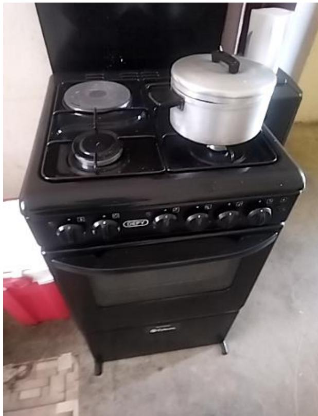
Figure 71: Example of Installed Hybrid Stove
