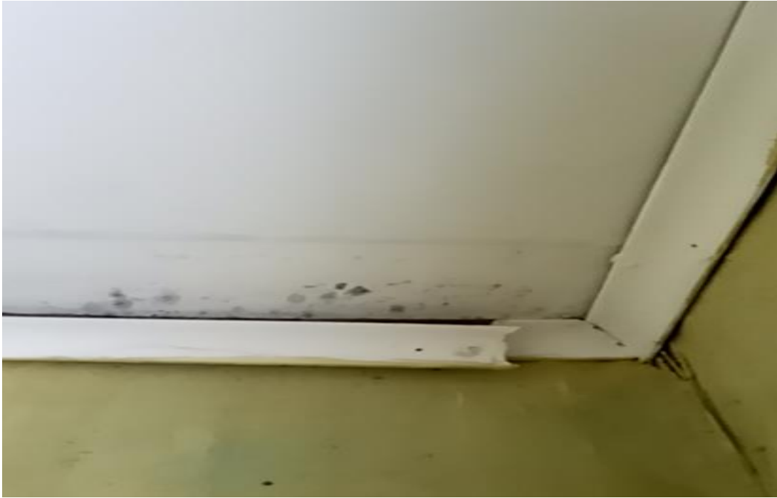
Figure 58: Loose cornice in a respondent's household
