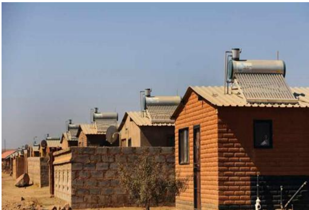
Figure 96: Solar panels and geysers
