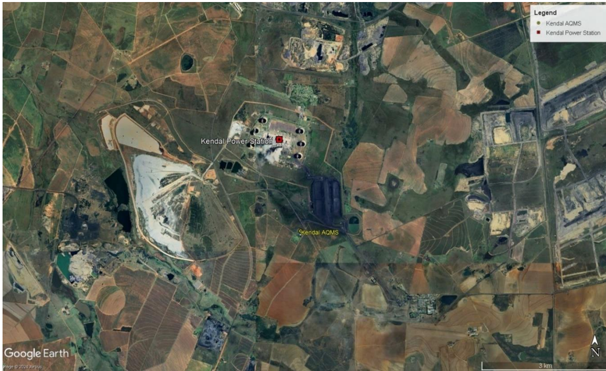
Figure 25: Map indicating the location of the Kendal AQMS relative to the Kendal power station
