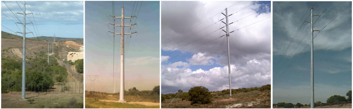
Figure 2.3: Examples of the proposed 132 kV monopole double circuit power line tower type.
