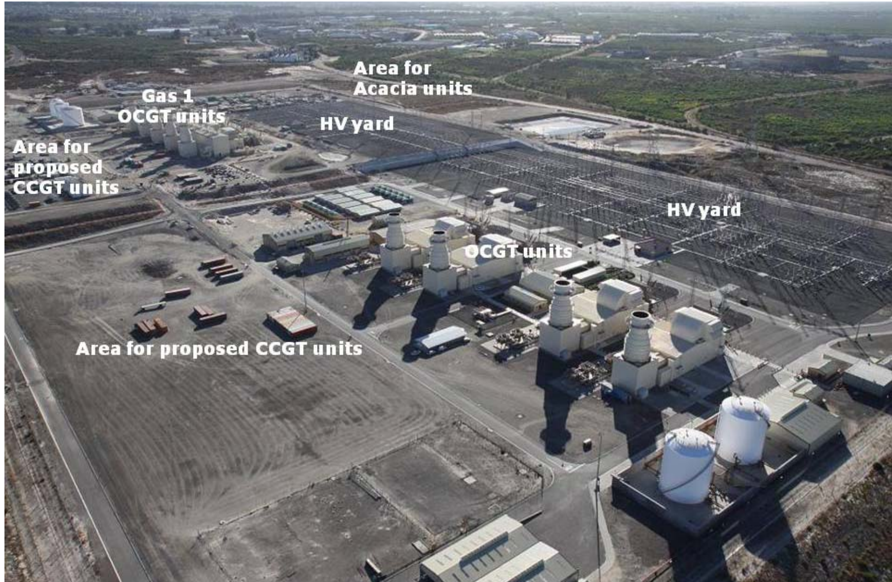
Figure 1.1: Aerial photograph of the Ankerlig Power Station site showing the existing power station infrastructure the power station expansion site, as well as the areas for the placement of Acacia and Port Rex gas units
