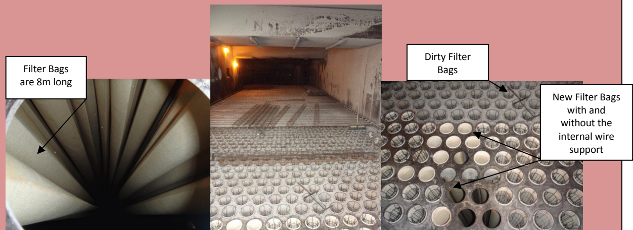
Figure 5: Inside a typical fabric filter plant
