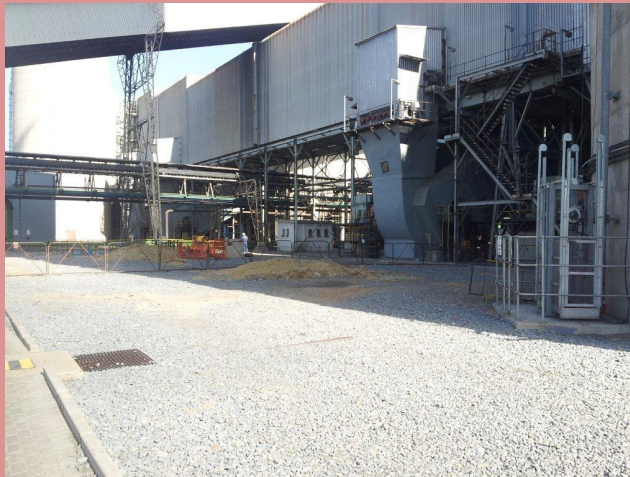
Figure 3: The area set aside for the construction of the proposed new compressor house (it is important to note that the entire area in the photo will not be utilised)
