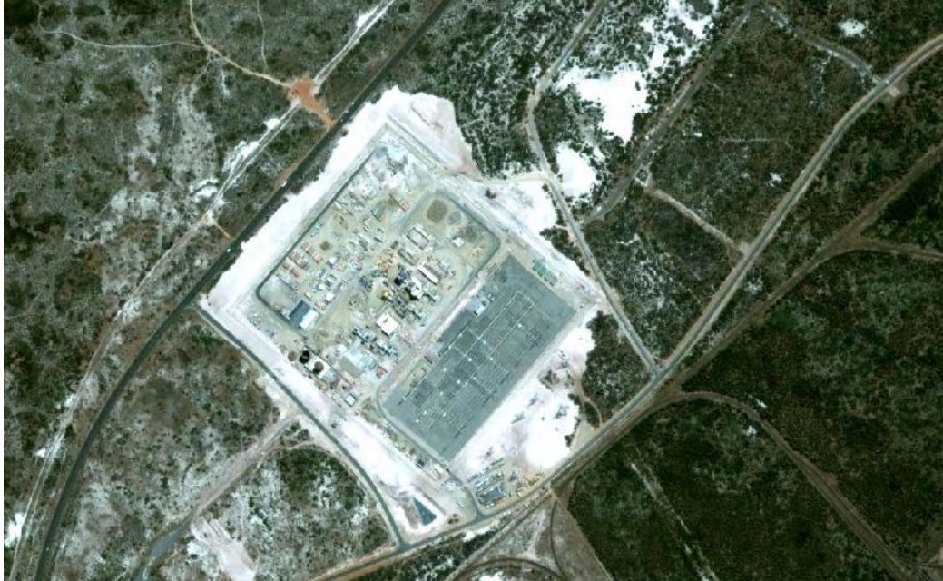
Figure 9.3: Aerial view of Atlantis OCGT (footprint 56 ha)
