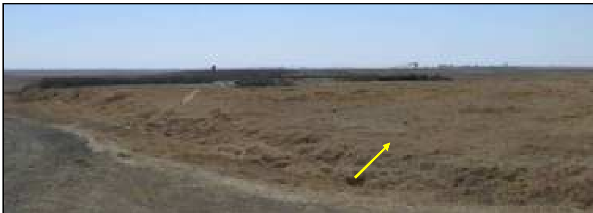
Figure 4-2: Existing waste disposal site with capped and rehabilitated area in the foreground
