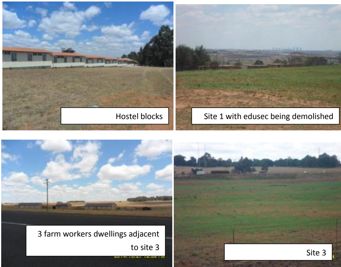
Figure 8: Photographs of Arnot Power Station, proposed sites and surrounds
