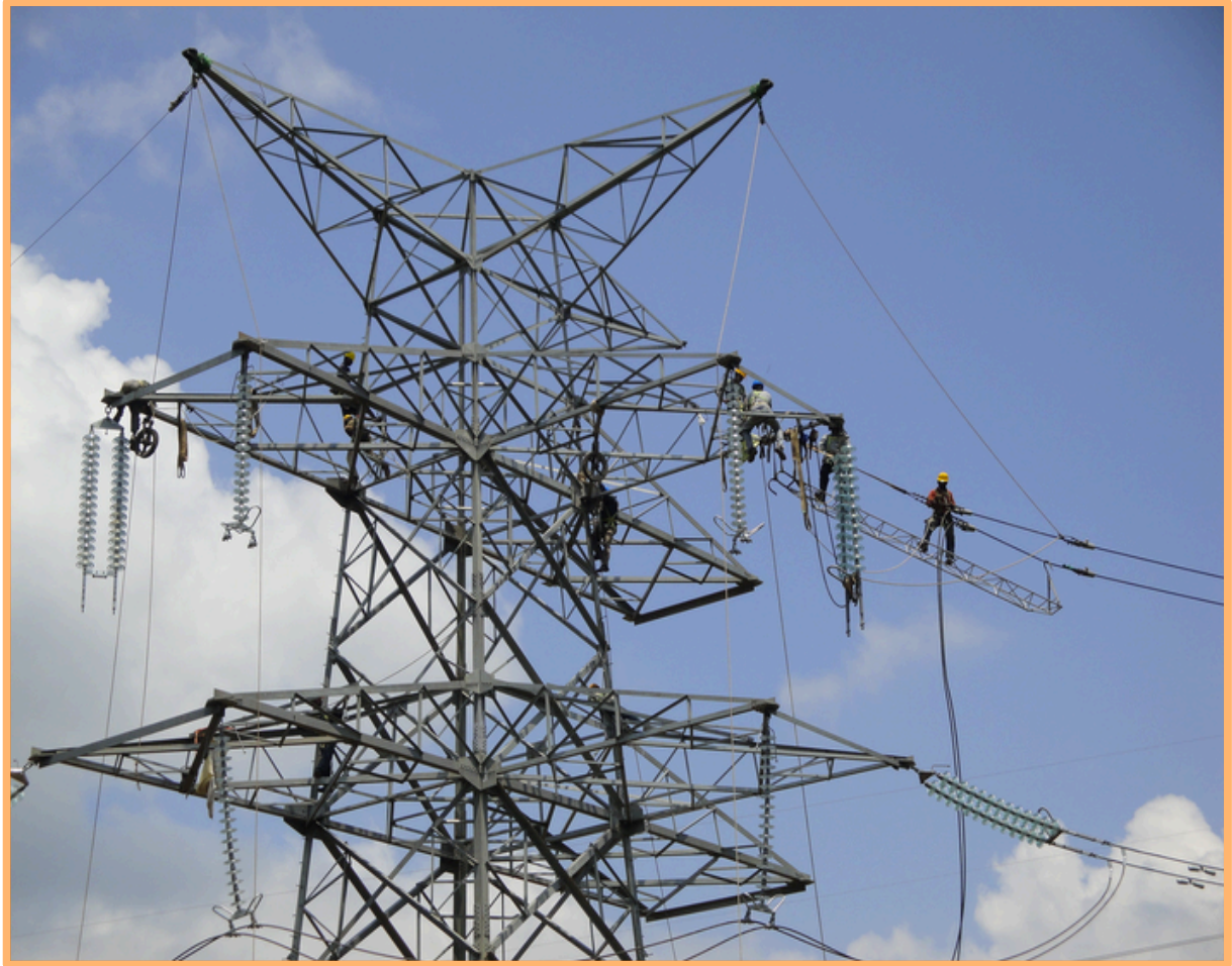
Plate 1: Shows the stringing of conductors for the power lines.
