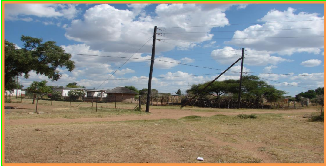
Plate 4: View of existing powerlines in the project area.
